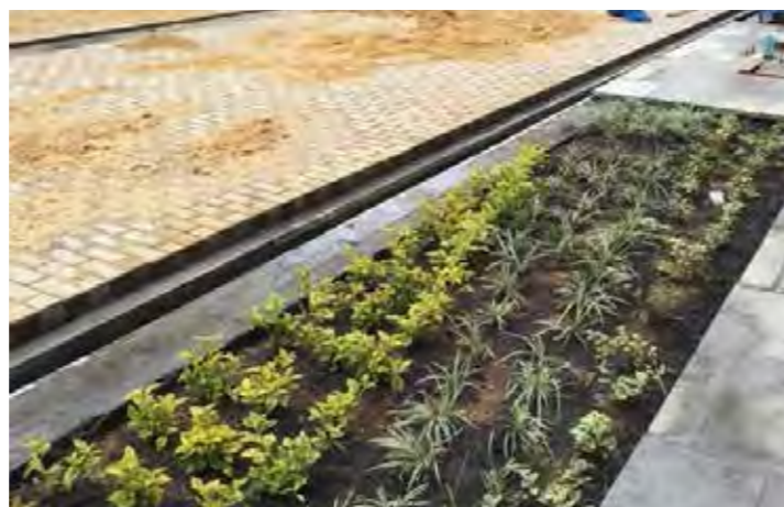
Figure 158. Paving treatment during construction - Source:SkyscraperCity
