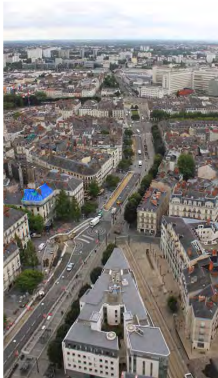
Figure 196. Remodelling work on the Cours des 50 Otages - Source: Llann Wé; Wikipedia Commons
