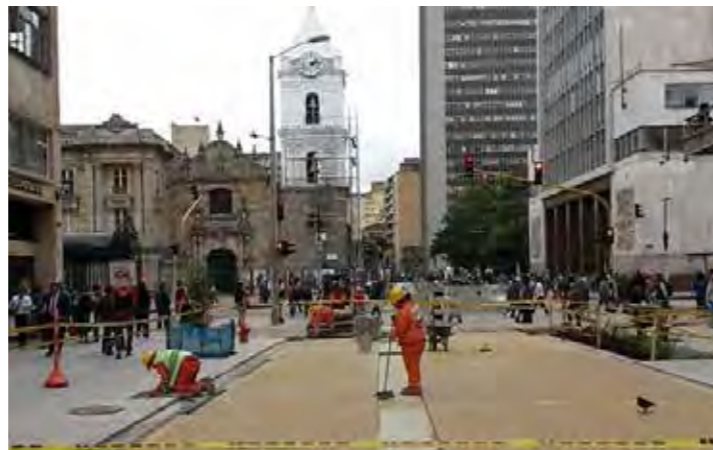
Figure 157. Pedestrianisation work on Carrera Séptima in Bogotá (Colombia) - Source:Wikimedia Commons
