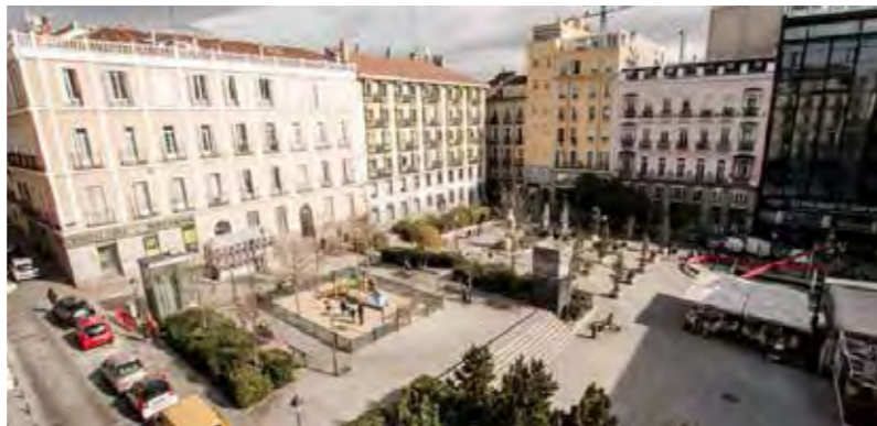
Figure 100. Plaza de Pedro Zerolo (formerly Plaza de Vázquez de Mella) following redesign - Source: Ayuntamiento de Madrid
